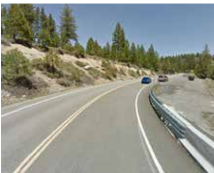
Existing pull-off location is not signed.
