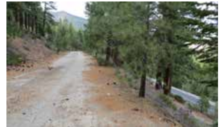
Existing condition along old highway 431.
