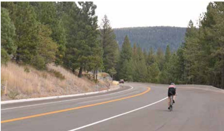
Adequate shoulder width for a bike lane exists along the highway from Incline Village to the summit.
