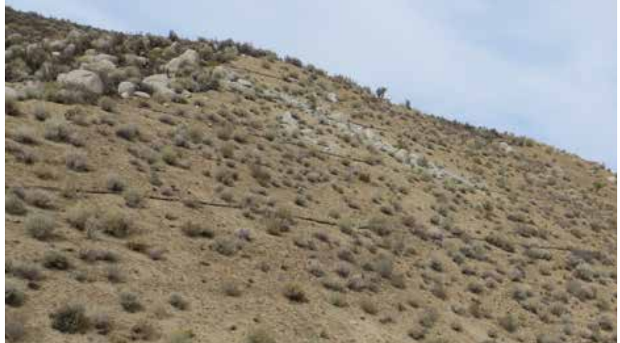
Naturalized rock cuts are preferred over the use of rock fall protection fencing.
