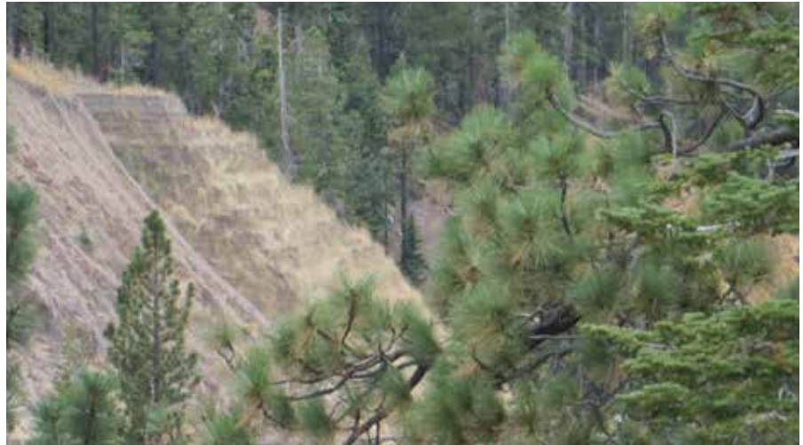
Terraced and planted rock cuts such as those used on US 50 in Lake Tahoe are preferred over the use of rock fall protection fencing.
