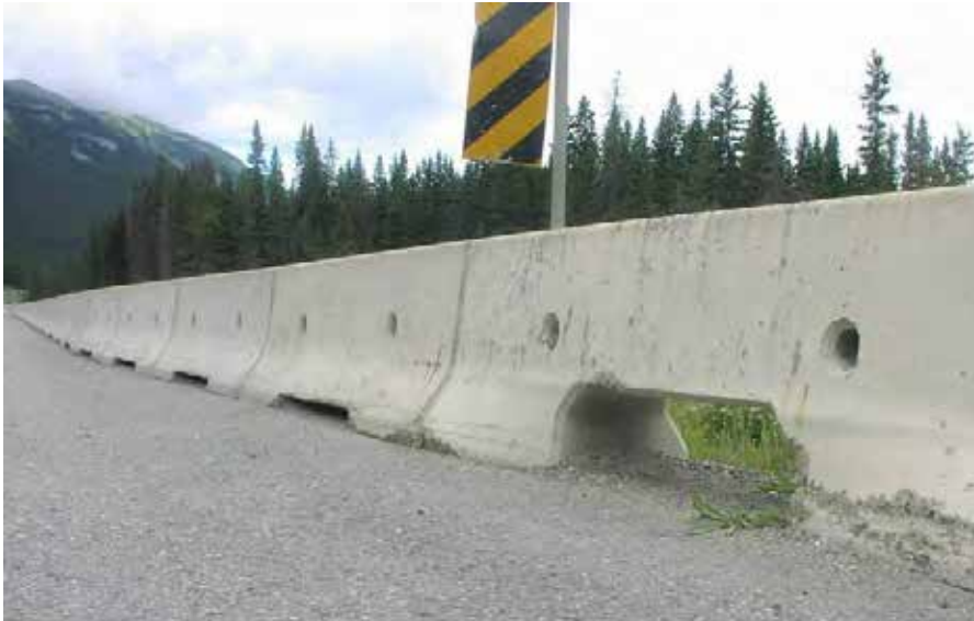
Barrier rails with scuppers installed at every fifth barrier facilitate small animal passage through the barrier according to a study by Caltrans.
