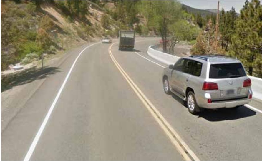
Emergency pull-off locations should be identified every one to two miles through the switchbacks east of Slide Mountain Road.
