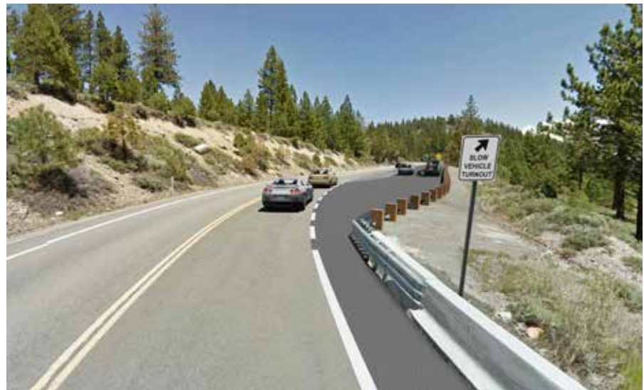
Traffic often queues behind slow-moving vehicles ascending the summit. Slow vehicle turnouts can be enhanced to improve traffic flow and create slow vehicle passing lanes where possible.
